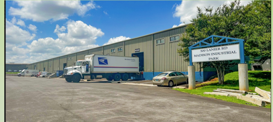
500 Lanier Rd – $9mm ($63/SF) 143,500 SF (3 Buildings) Jetplex/Madison Industrial Market
