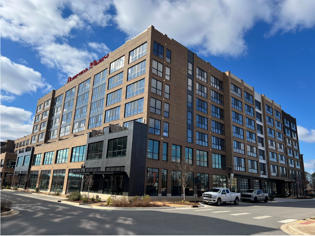
Anthem House at MidCity – Hotel & Apartments
